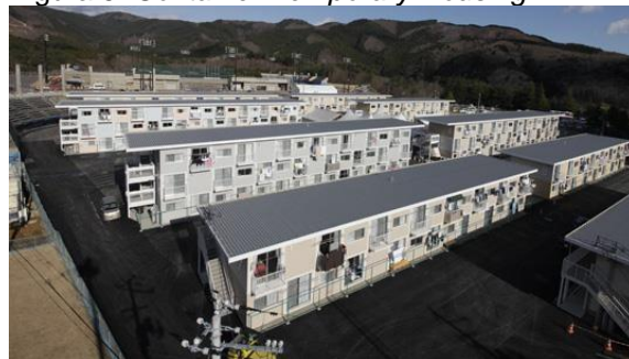
Figura 5: Container Temporary Housing .
