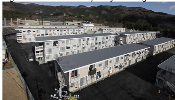
Figura 5: Container Temporary Housing .
