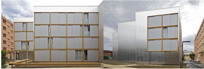
Figura 2. 50 Modular Timber Apartments. Fonte: PHILIPPE RUAULT.
