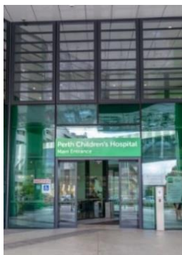
Figura 12: Entrada Principal do Perth Children's Hospital
