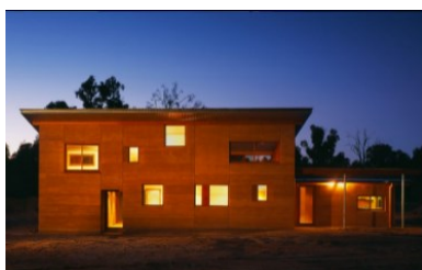
Figura 35: Butterfly Residence - Taipa mecanizada
